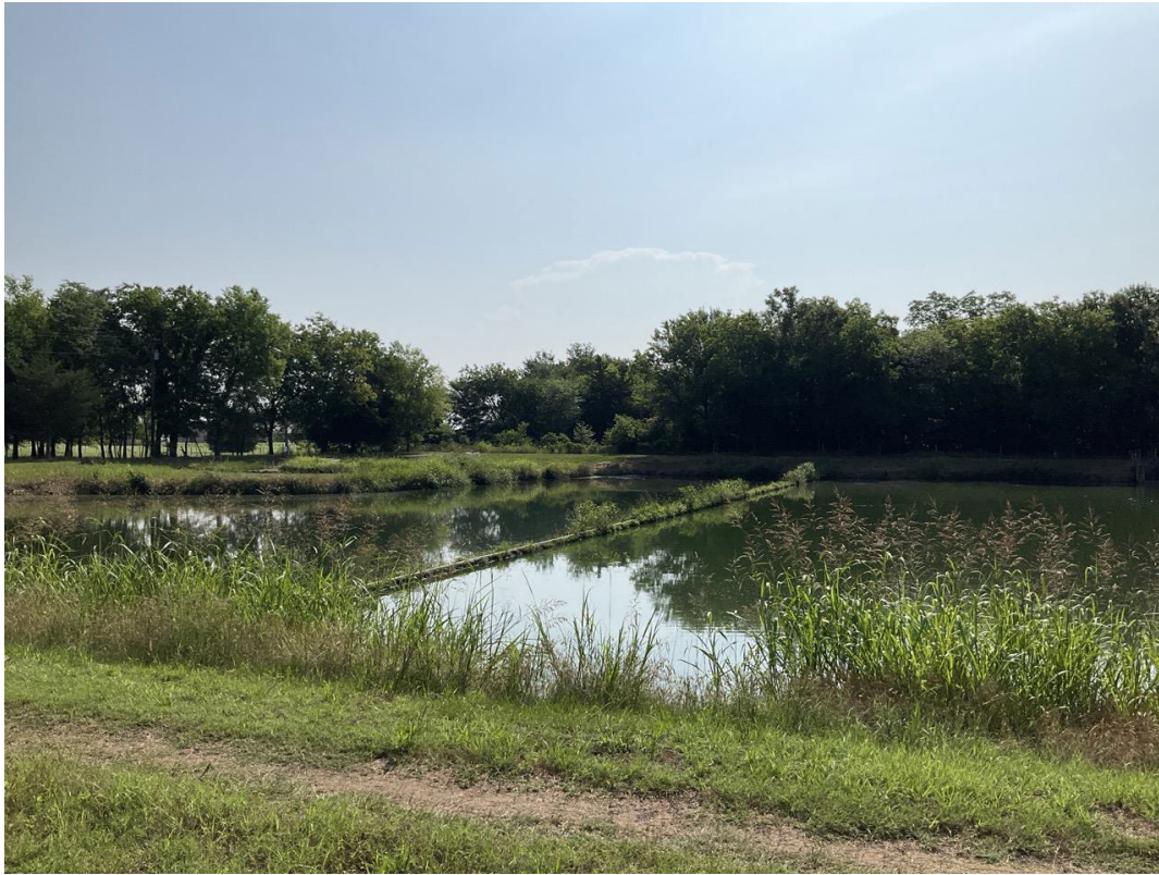
Photo 03: View of Map Key 1, western water treatment facility.
