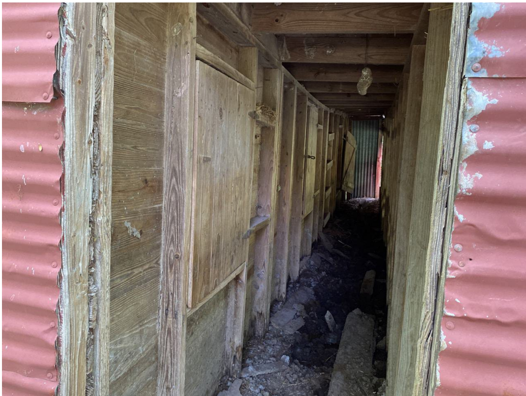
Photo 14: Interior of old barn viewing from the entrance.
